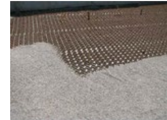
GRAVELPAVE2 DURING INSTALLATION
