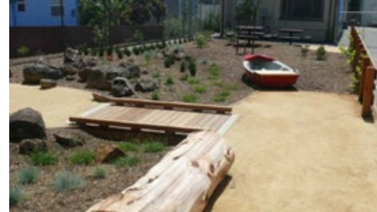
A STABILIZED DECOMPOSED GRANITE THRESHOLD, FENCING AND AN EMBEDDED LOG HELP TO KEEP MULCH CONTAINED.
